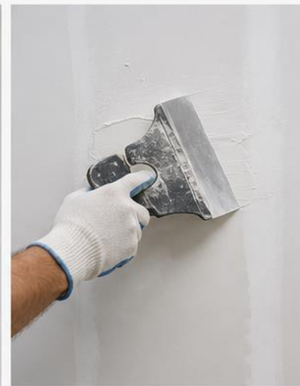
2. SKIM COATING AND FINISHING
